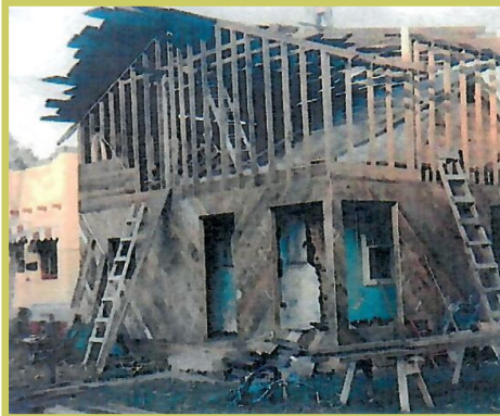
Ongoing remodeling at the Nequette house (Jan Nequette)
